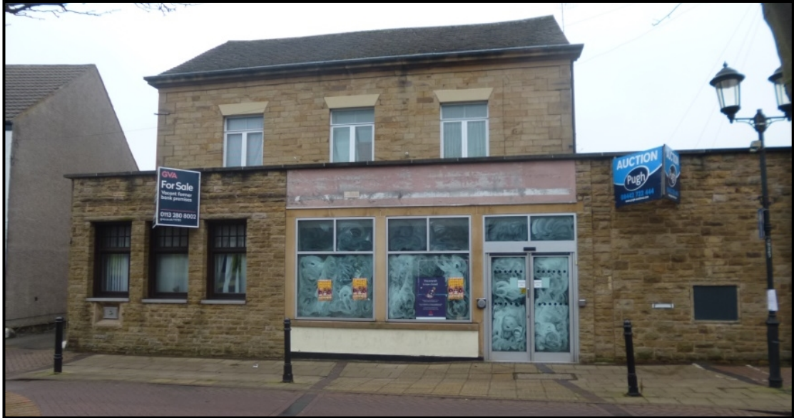
Above: The application site
